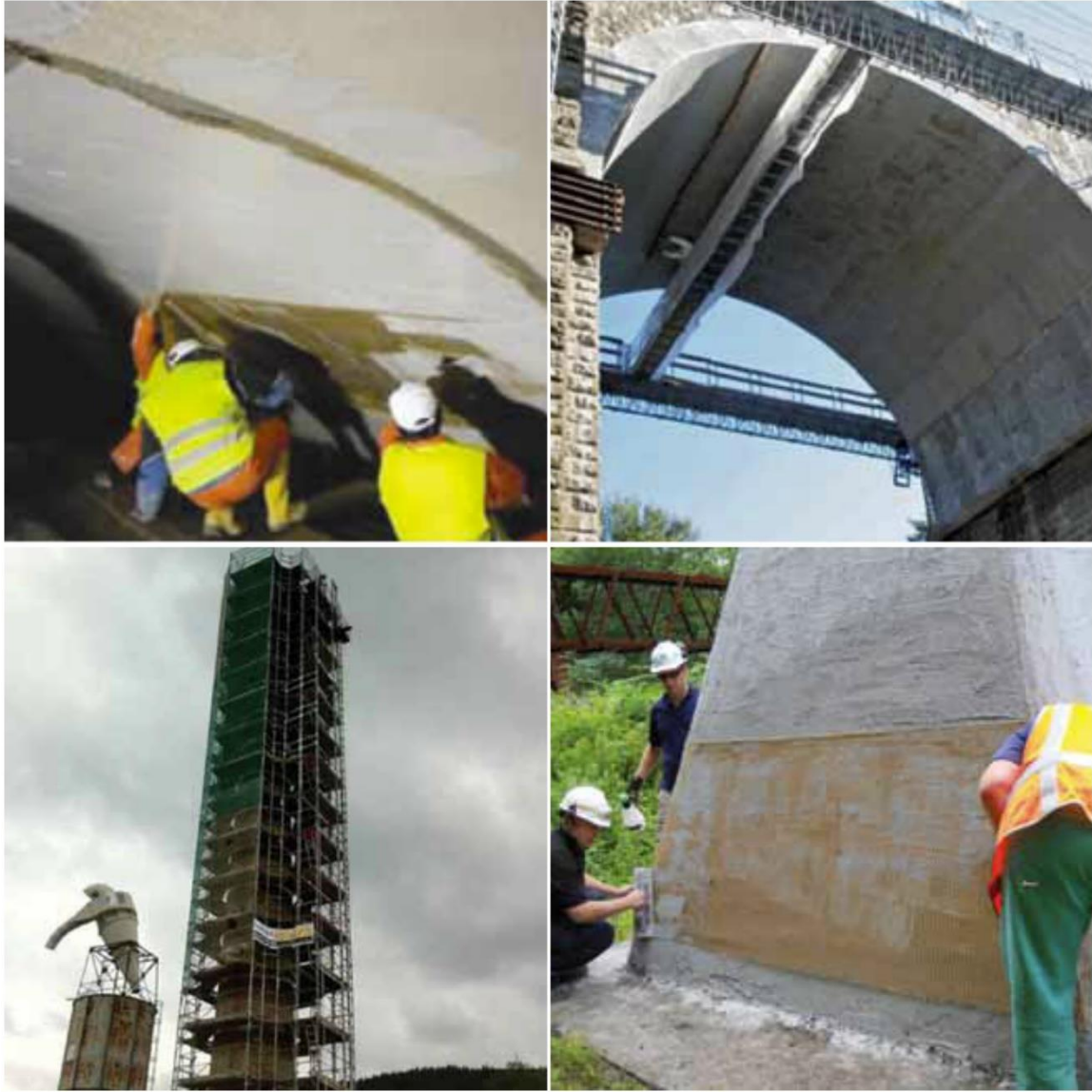
Figure 1.1 (1) Tunnel lining with PBO-FRCM in Greece, (2) chimney strengthening with carbon FRCM in France, (3) railway bridge strengthening with PBO-FRCM in Italy, and (4) Concrete railway bridge pedestal strengthening with PBO-FRCM in northern New York (Nanni 2012).
