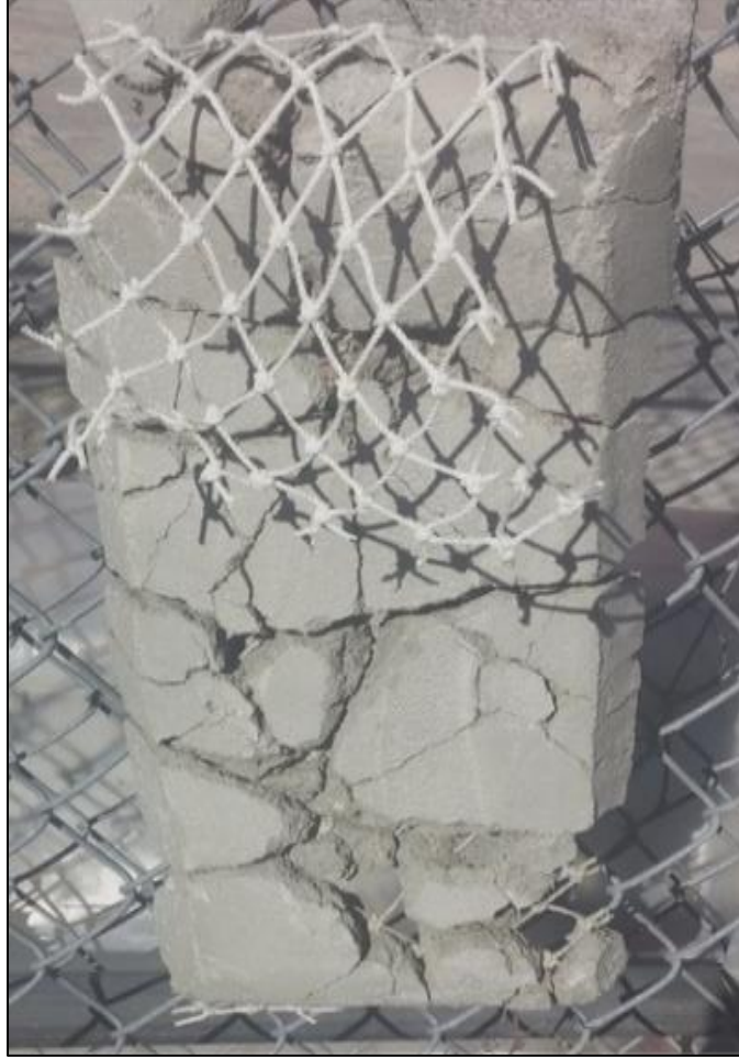
Figure 2.4 Crushed mortar with embedded FN reinforcement.
